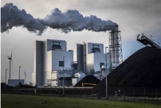
RWE's power station in Eemshaven uses both coal and biomass as fuel. © ANP / Kees van de Veen
